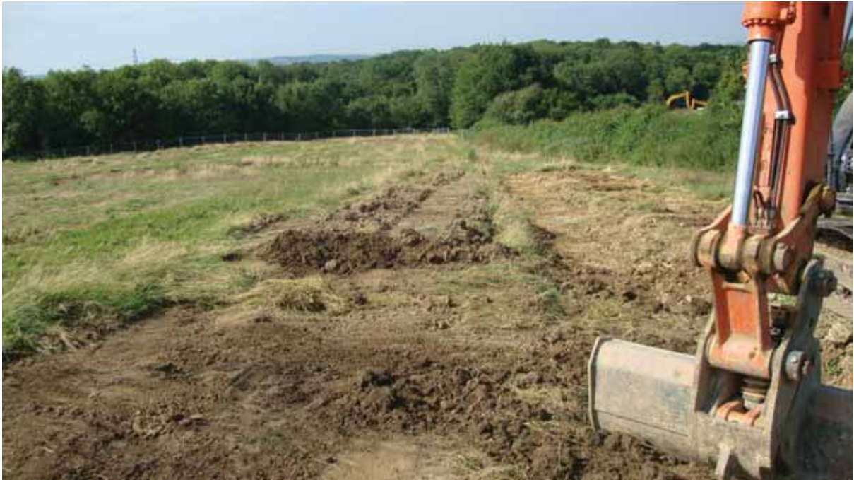
Plate 166: Backfilling of the trench 22 in field 3
